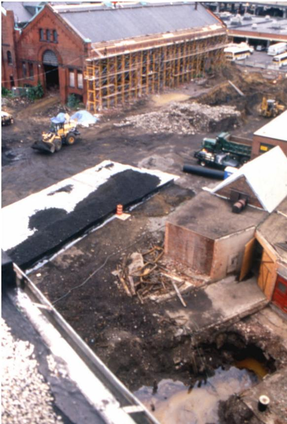
The picture on the left shows the excavations where underground structures and contaminated soils were removed.
