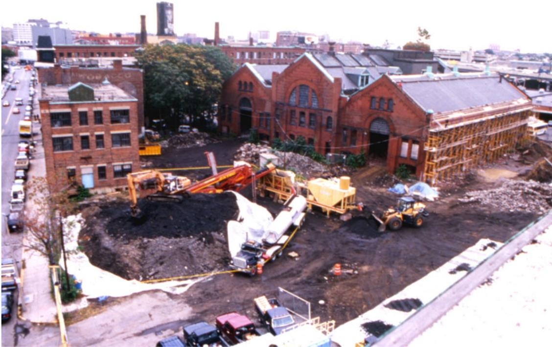
Screened material was conveyed on a belt to a pugmill (yellow). Computer controls on the pugmill ensured the proper amount of cement is added and mixed into the contaminated soils. The mix design for this site required a 6% addition of cement. Treated material exits the pugmill on another belt conveyor. The treated material was staged on plastic sheeting for curing and treatment performance verification.
